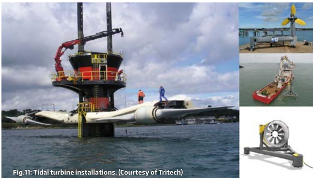
Fig.11: Tidal turbine installations. (Courtesy of Tritech)
